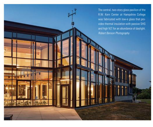
associate director with Atelier Ten, "Various glazing types were studied throughout design from triple glazing to high-performance, double-glazed units. The building was constructed using double-glazed, low-e units with a U-value equal to .28 and SHGC equal to .40 for the northern orientations and U-value equal to .29 and SHGC equal to .30 for all other orientations."
